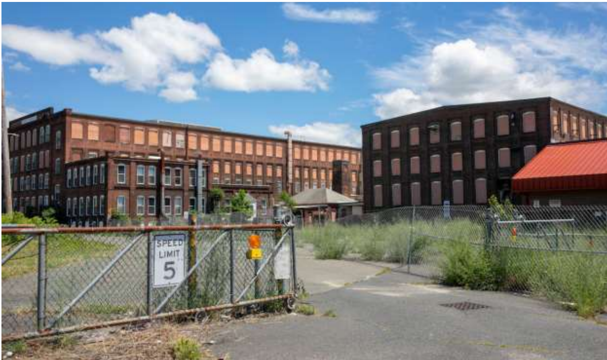
The site of the defunct Hampden Papers Inc. at 100 Water St. in Holyoke, where the Boston based Chestnut River Power and Infrastructure is proposing the construction of a $200 million data center. (Michael J. Fiedler / Special to The Republican)Michael J. Fiedler / Special to The Republican
